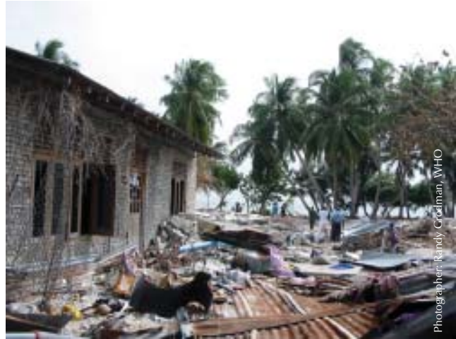
Damage and destruction caused by the passage of the Tsunami in the Maldives.
