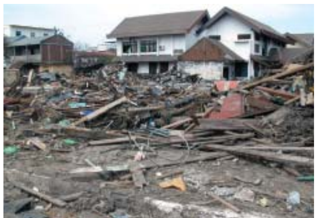
Damage caused by the Tsunami in Banda Aceh in Indonesia.
