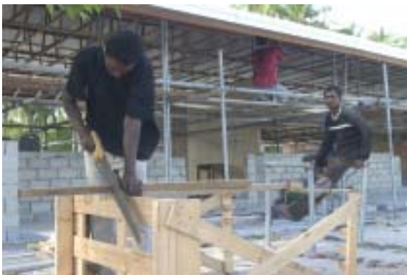
Reconstruction underway in the Maldives.
