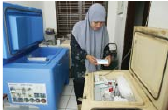
Cold chain used for vaccine and supply storage and health facilities.
